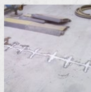
Crack stitching
