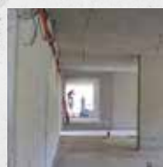
Large surface restoration
