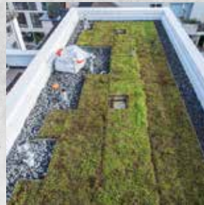
Under ballast / green roofs
