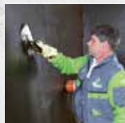
Waterproofing against Radon
