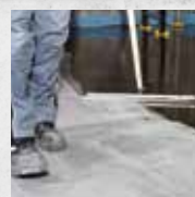
Coating after 24 hours
