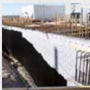
External basement waterproofing
