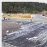
Floor slab waterproofing
