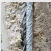
Corrosion protection (coating)
