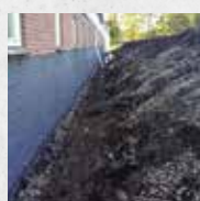
External basement waterproofing
