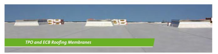
KÖSTER TPO Roofing Membranes can be installed by mechanical fastening, loose laying, or full surface adhesion on flat or green roofs. They stand out due to their excellent application and outstanding mechanical properties as well as through their durability and sustainability. KÖSTER produces both thermoplastic polyolefine (TPO) and ethylene copolymer bitumen membranes. The standard color of KÖSTER TPO Membranes is light grey, for ECB Membranes the standard color is black.
